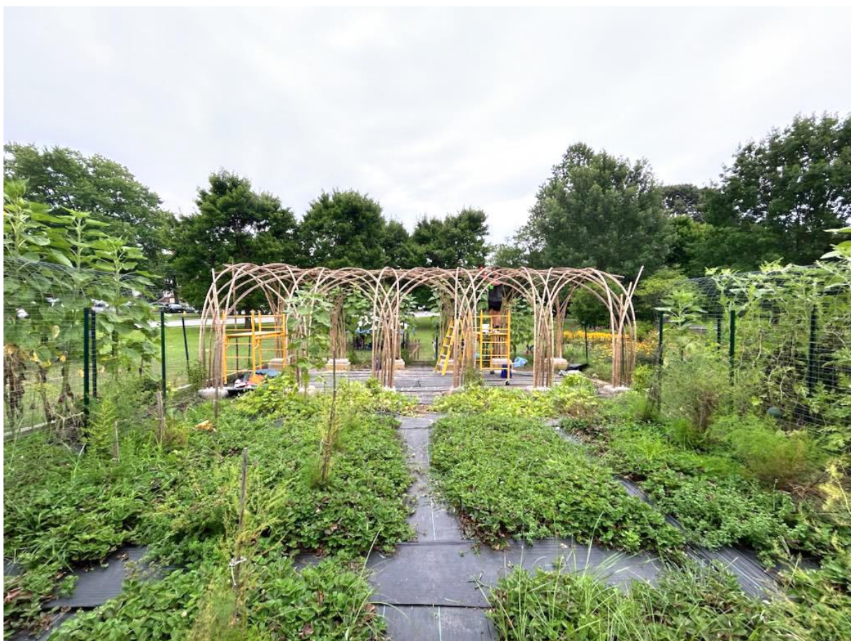
Farmunity Pavilion – SOS (work-in-progress)
